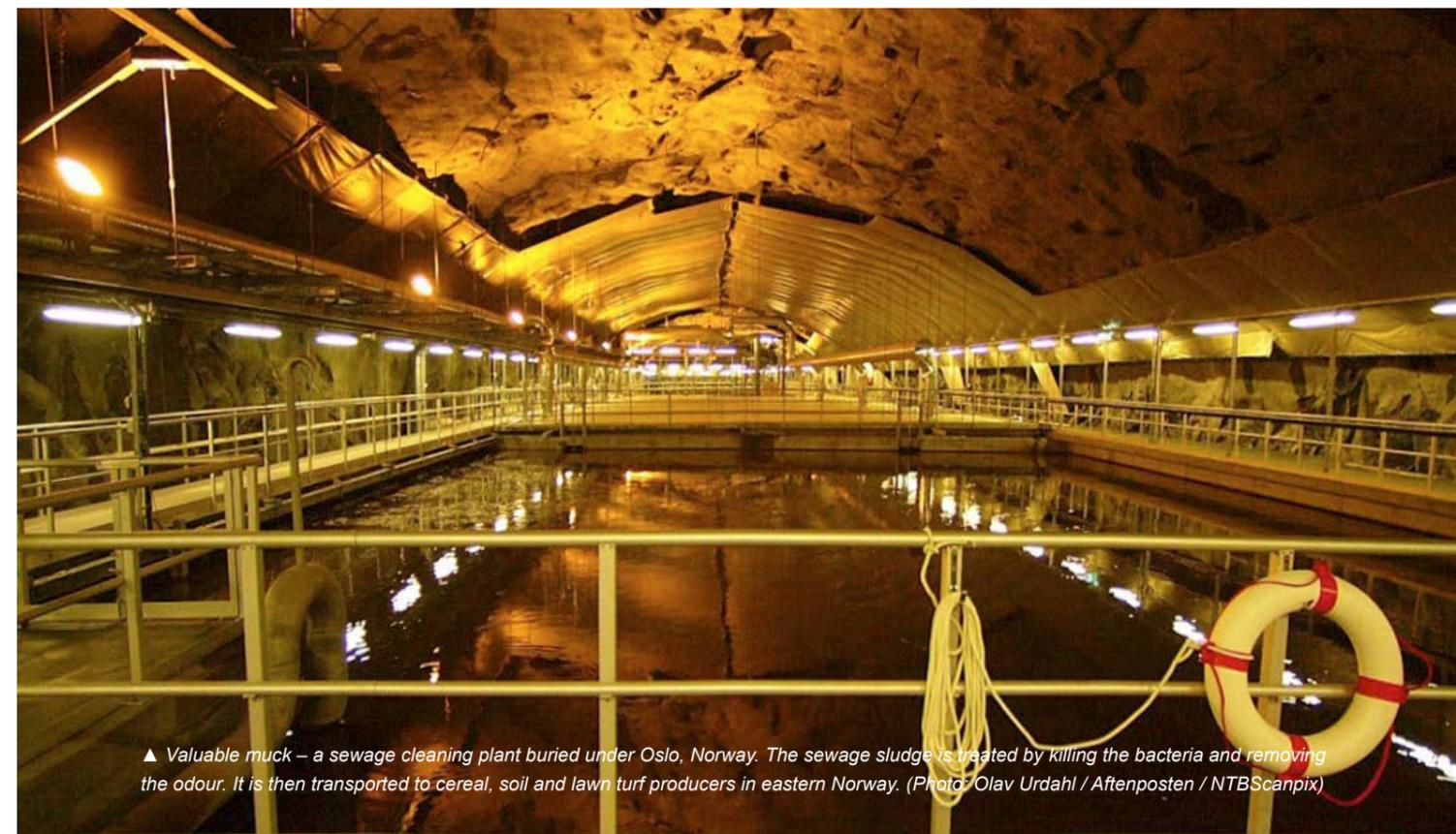
▲ Valuable muck – a sewage cleaning plant buried under Oslo, Norway. The sewage sludge is treated by killing the bacteria and removing the odour. It is then transported to cereal, soil and lawn turf producers in eastern Norway. (Photo: Olav Urdahl / Aftenposten / NTBScanpix)
